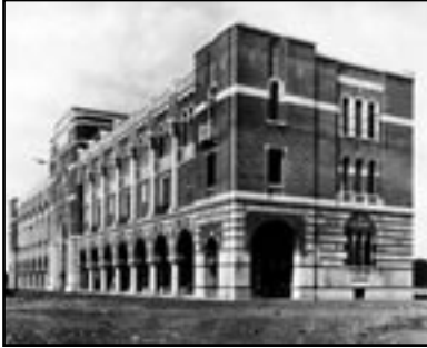
Rice Administration Building
